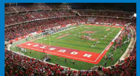
UNIVERSITY OF HOUSTON - TDECU STADIUM
