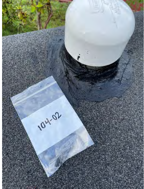
Photo #10: Roofing mastic at shed roof penetrations, (material 104).
