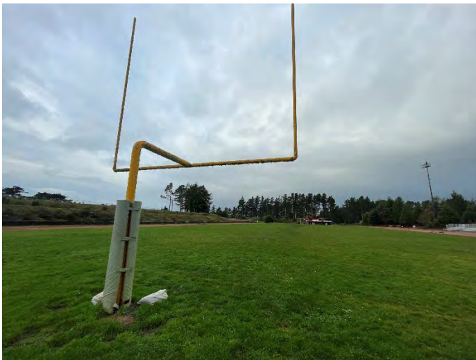
Photo #3: Goal post on east side of football field, yellow paint on metal, sample Pb02.
