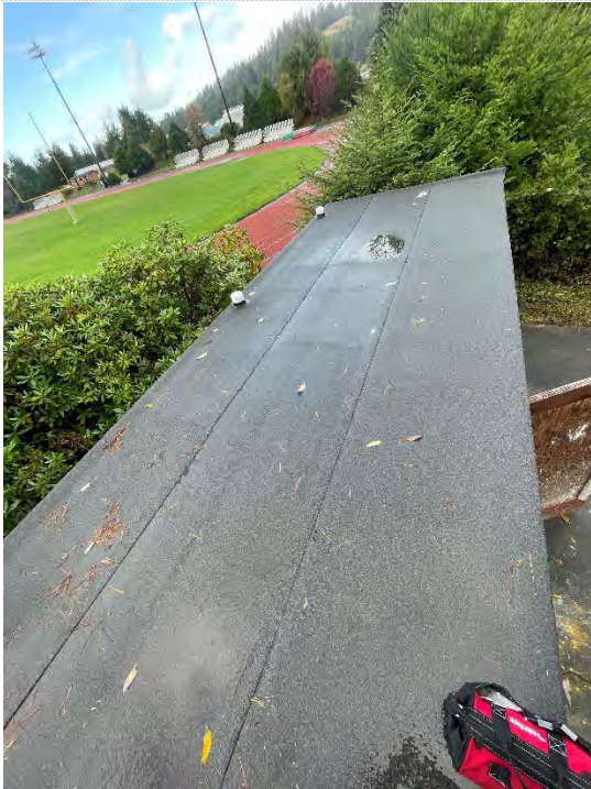
Photo #9: Rolled composition roofing on equipment shed.
