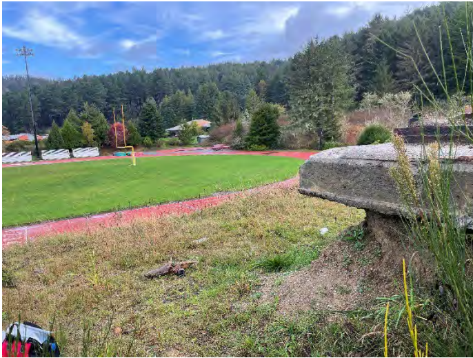
Photo #5: Two former high mast lighting concrete bases, south side of track and field.
